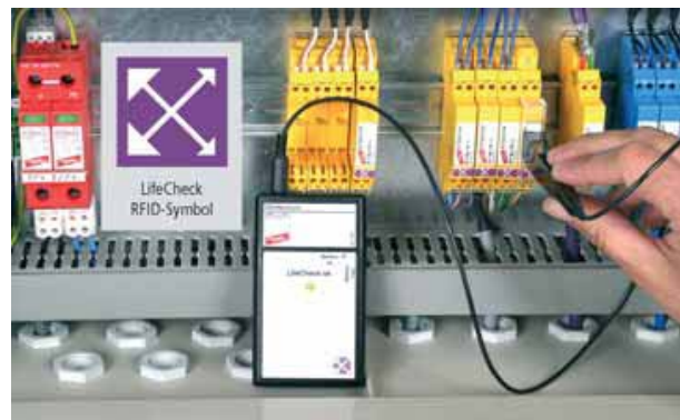
Fig. 1. Testing an SPD module with RFID system (LifeCheck).
